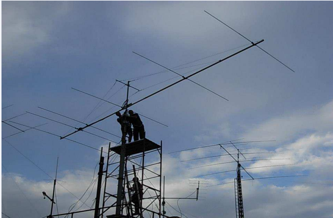
Installing antennas at Monte Pellegrino (IR9Y) by IT9RGY
